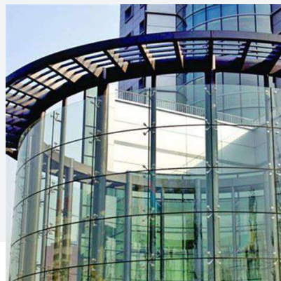
Project:U.K curtain wall
